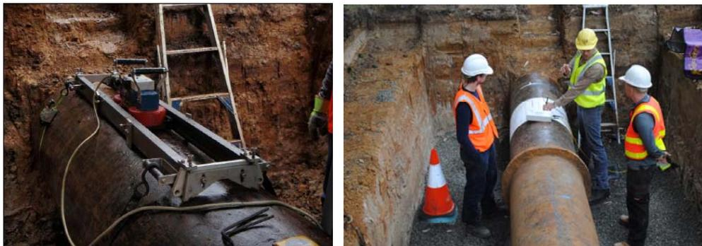
**Figure 7.** MFL tool in Pit 1 (left) and BEM grid (right).
