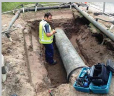
Figure 1. Collecting soil and other data at an open pit in the Hunter Water network (Photo courtesy of Hunter Water)
